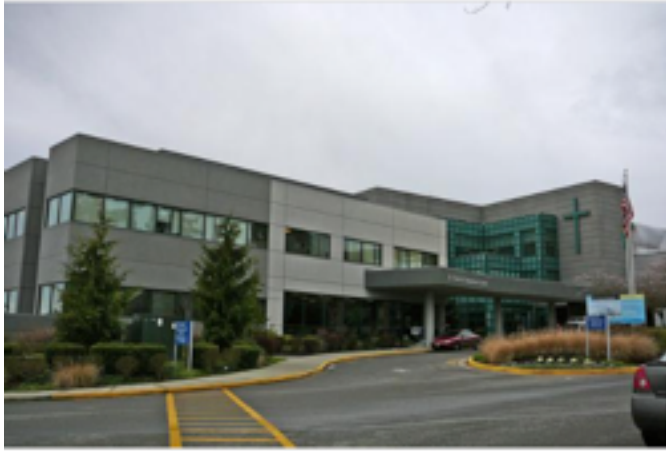
St Francis Hospital 1987
