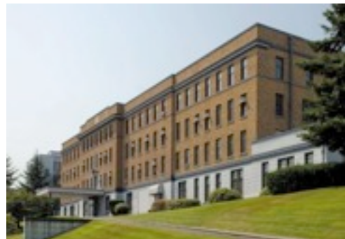
Pierce County Hospital 1929
